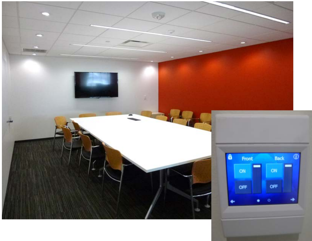
Figure 21: Conference room and associated digital controller.
