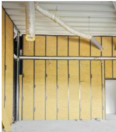
Examples of Cavity Insulation and Continuous Insulation respectively 3
