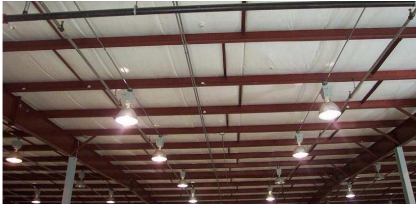
Figure 4. Roof Insulation in Metal Buildings 2
