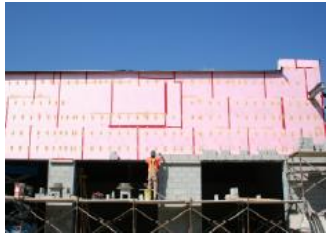
Examples of Cavity Insulation and Continuous Insulation respectively 3
