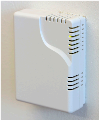
Figure 2: Carbon dioxide sensor
