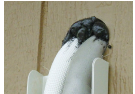
Figure 2 Air seal and waterproof wall penetrations.
