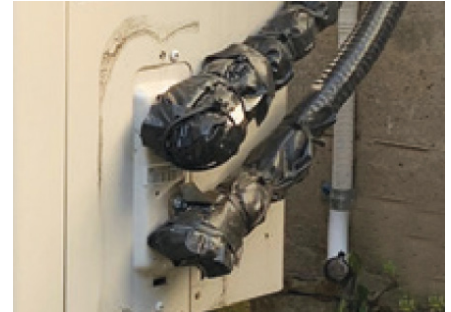
Figure 1 Insulate and tape flare nuts to prevent cracks due to frost formation.
