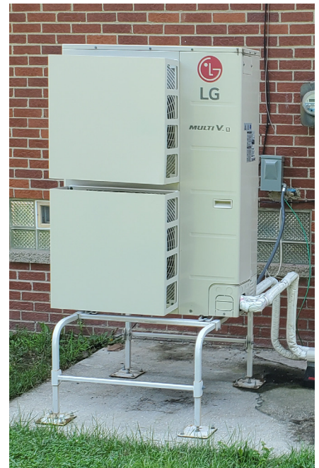
Figure 4 Proper placement: Away from drip line, on stand, with wind baffle and insulated line set.
