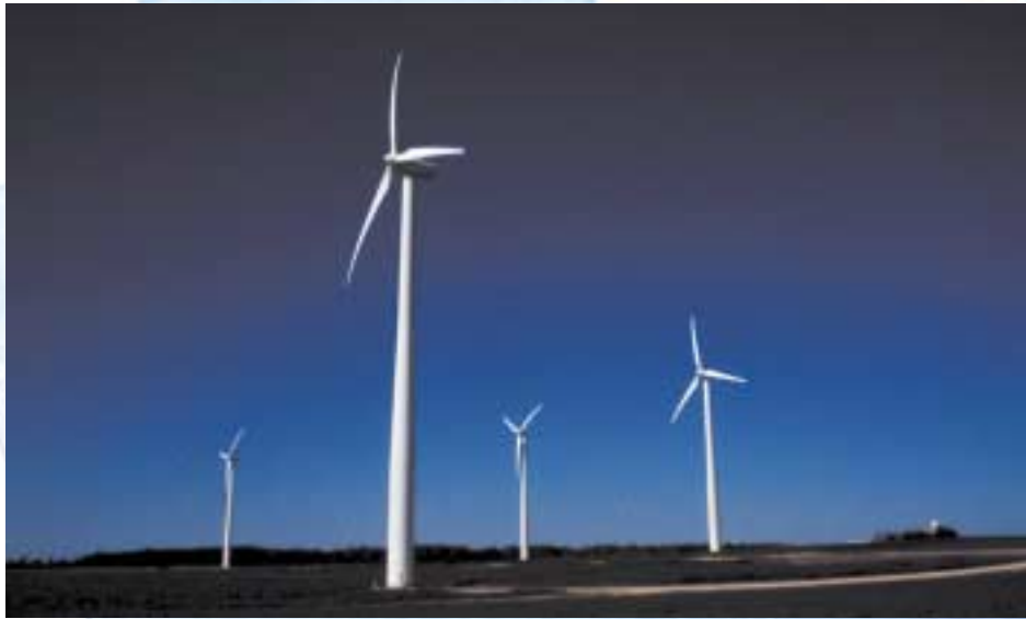
Four Vestas wind turbines rise 292 feet above farmland in Kewaunee County, Wisconsin, part of a 33 turbine wind farm shared by Wisconsin Public Service Corporation and Madison Gas & Electric Company.
