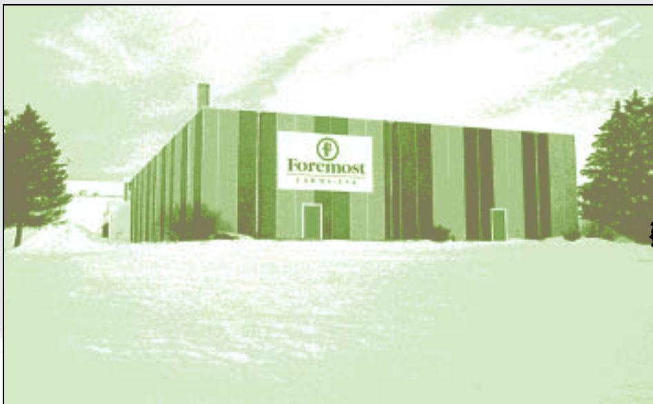
Cheese plant in Marshfield, Wisconsin, where UW-Madison scientists are testing ways to reduce the energy costs of producing cheese and whey.
