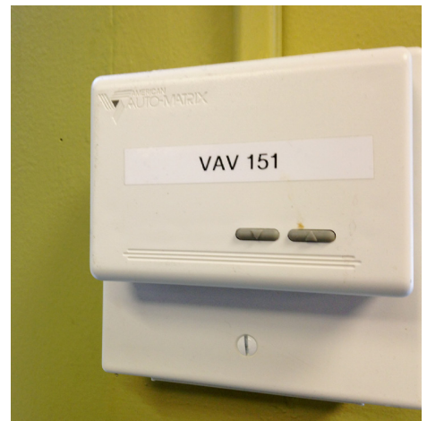
(Top) The fitness center is infrequently used, making controls effective. (Middle) Locker rooms were included in both lighting and HVAC control. (Above) The building's VAV system utilizes the sensing to turn down individual zones when nobody is present.
