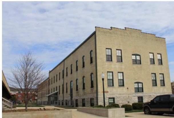
Figure 6. One of two Tobacco Lofts buildings.
