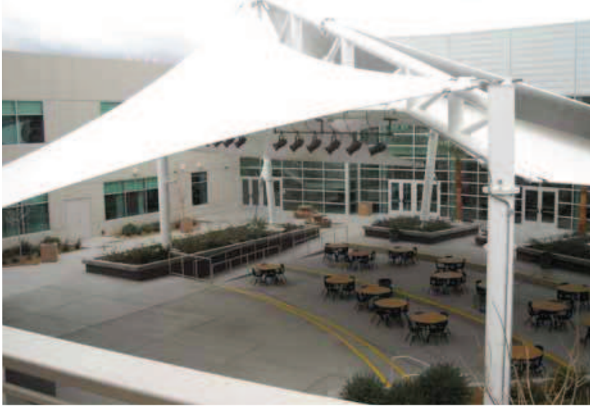
Courtesy of SH Architecture
